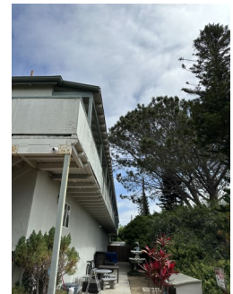
Star pine towering over Crescent Bay Inn 2nd story egress.
